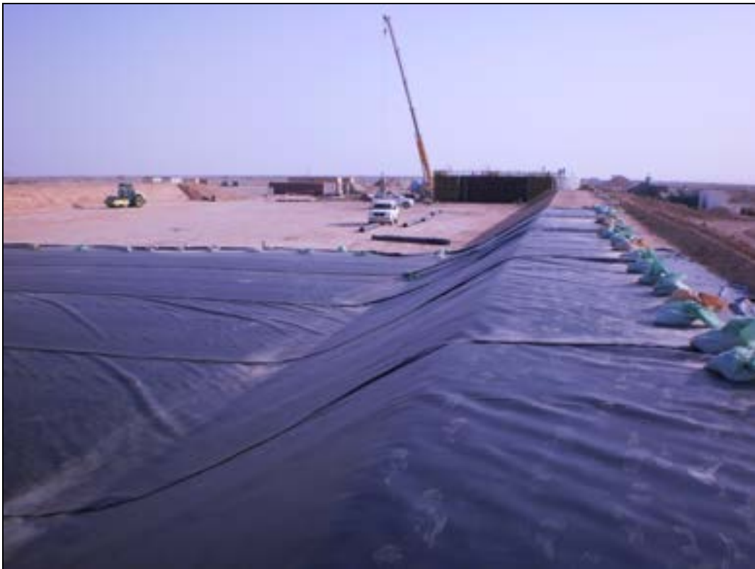
Installation of a HDPE liner in the buffer pond area
