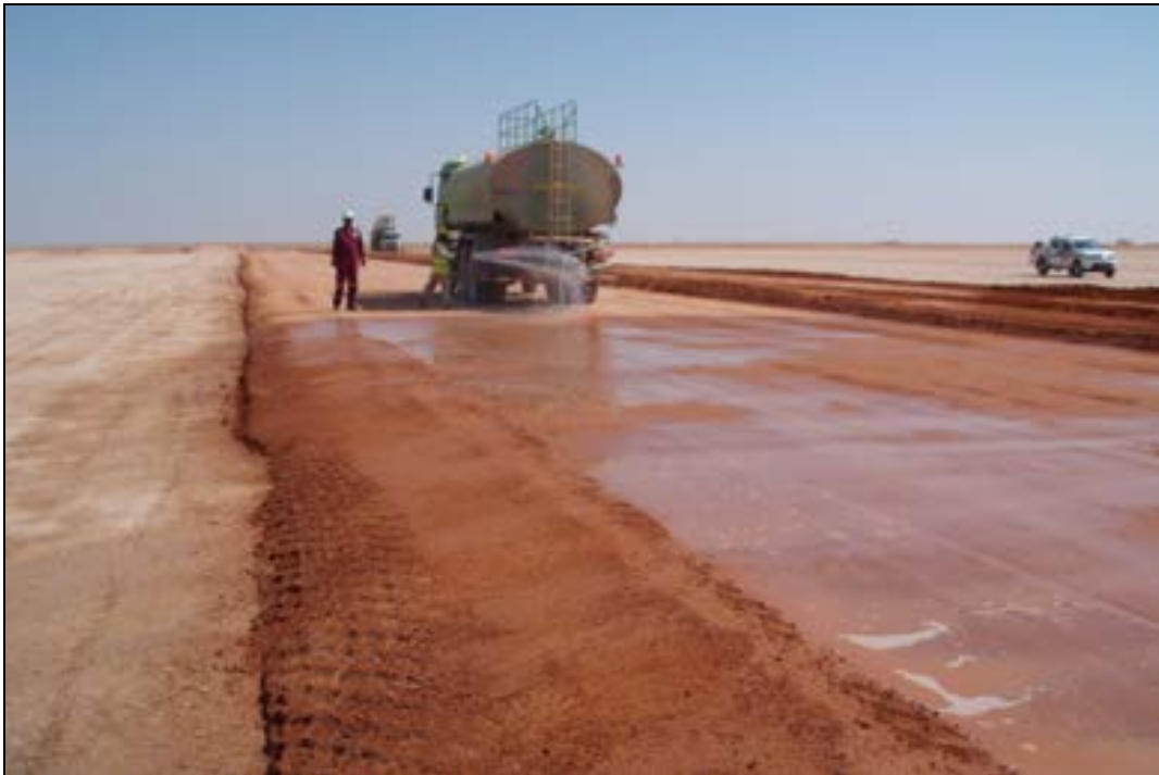
Installation of a mineral sealing layer
