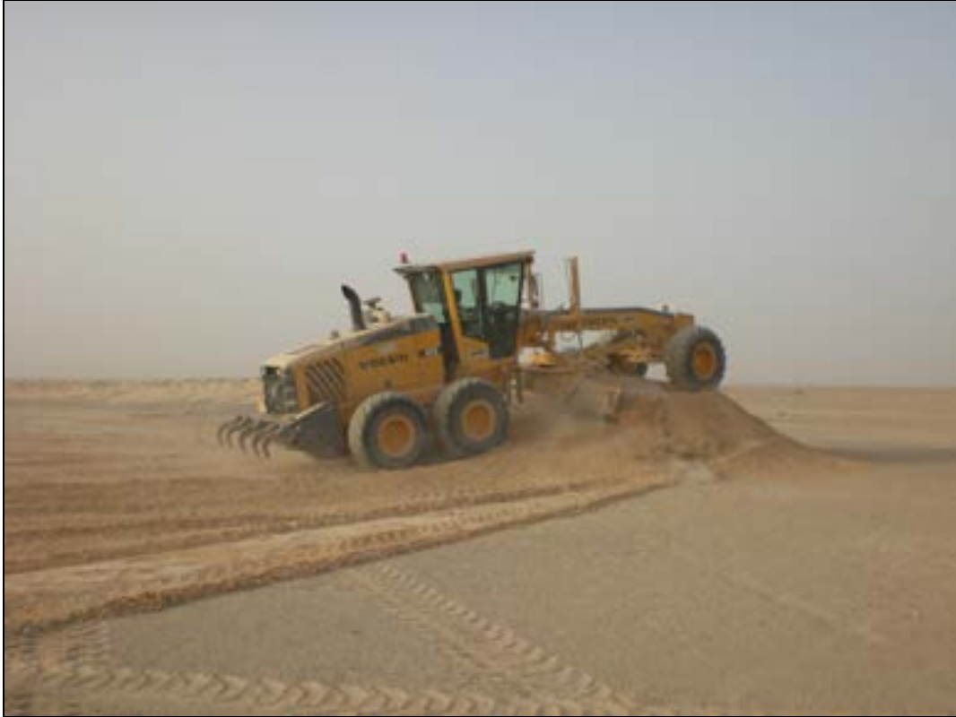
Start of the levelling works on site
